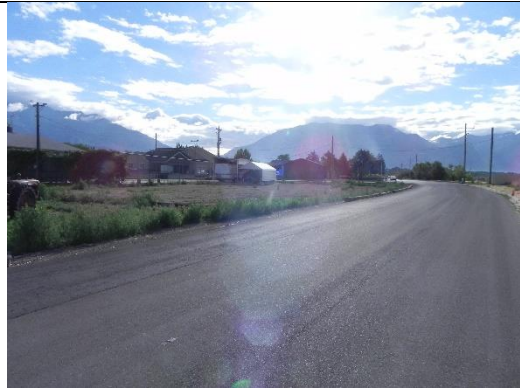
400 South looking east toward the intersection
