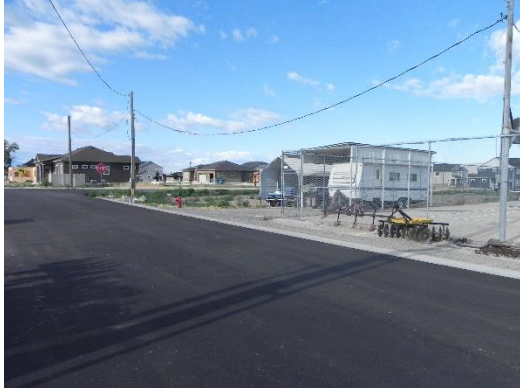
Holdaway Road looking southwest
