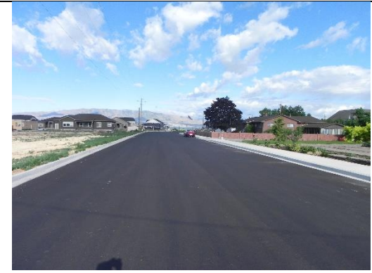
400 South looking west toward the intersection
