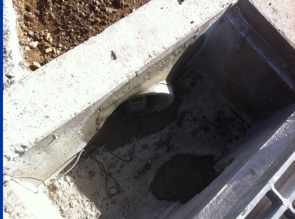
Storm Drain tie in west side of 900 West
