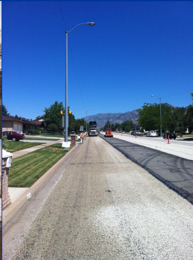
Medical Drive 500 West Crack Seal Chip Seal
