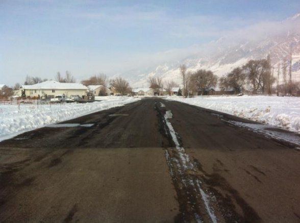
450 West SR13 New Road Sidewalk
