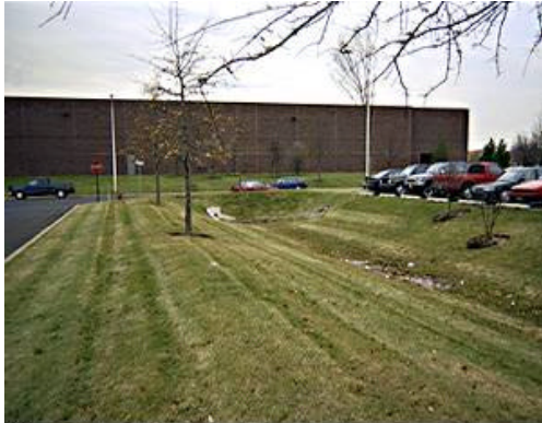
Grassed swales can be used along roadsides and parking lots to collect and treat storm water runoff
