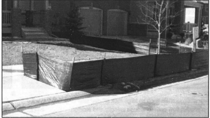
■ Silt fence can be used to keep sediment on the property.
