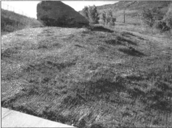
■ Erosion control blankets help stabilize slopes, retain moisture for seed germination, and reduce wind erosion.
