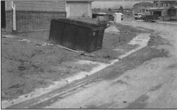
■ This site is in violation because sediment is not being contained on the jobsite.
