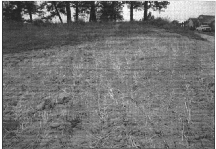
■ Crimp mulch perpendicular to slope.
