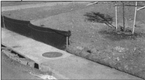
■ This site is in violation because sediment is not being contained on the jobsite.
