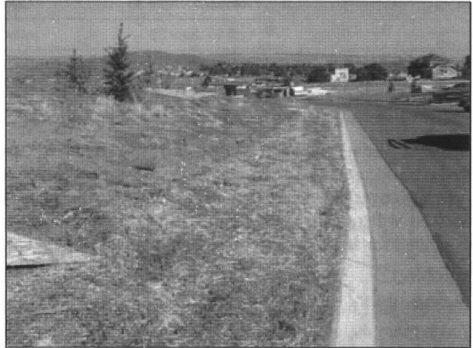
■ Erosion control blankets can be used along a sidewalk or street edge to help grass create a stable buffer strip.
