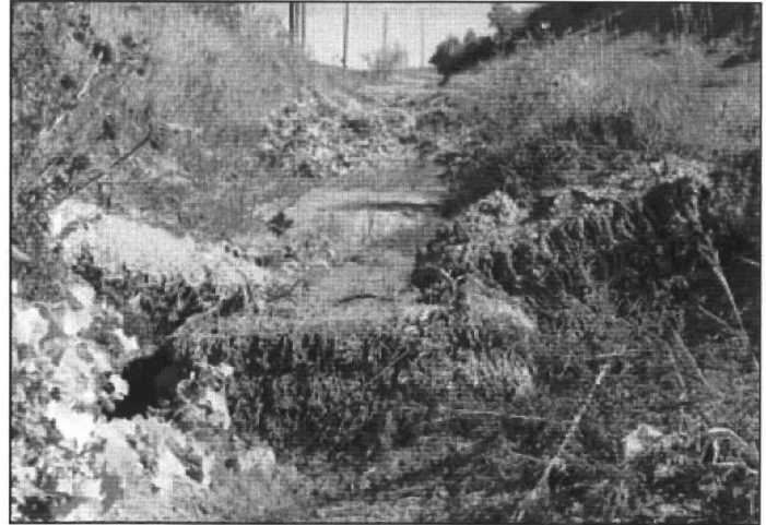
■ Straw bales or rock check dams must be wider than the flow path with a low point in the middle for overflow.
