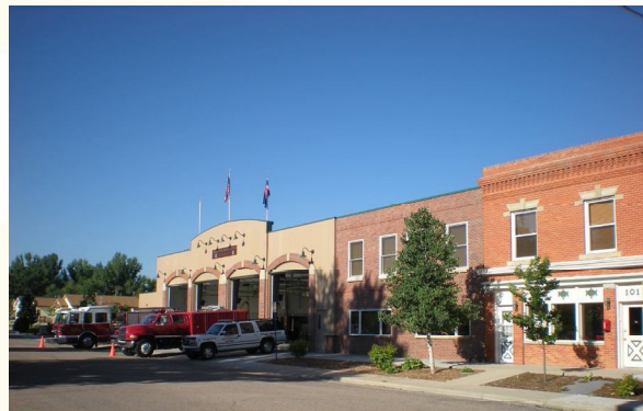
Milliken Fire Protection District Station #1
